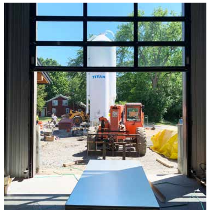
Using sustainable and repurposed materials was paramount.
